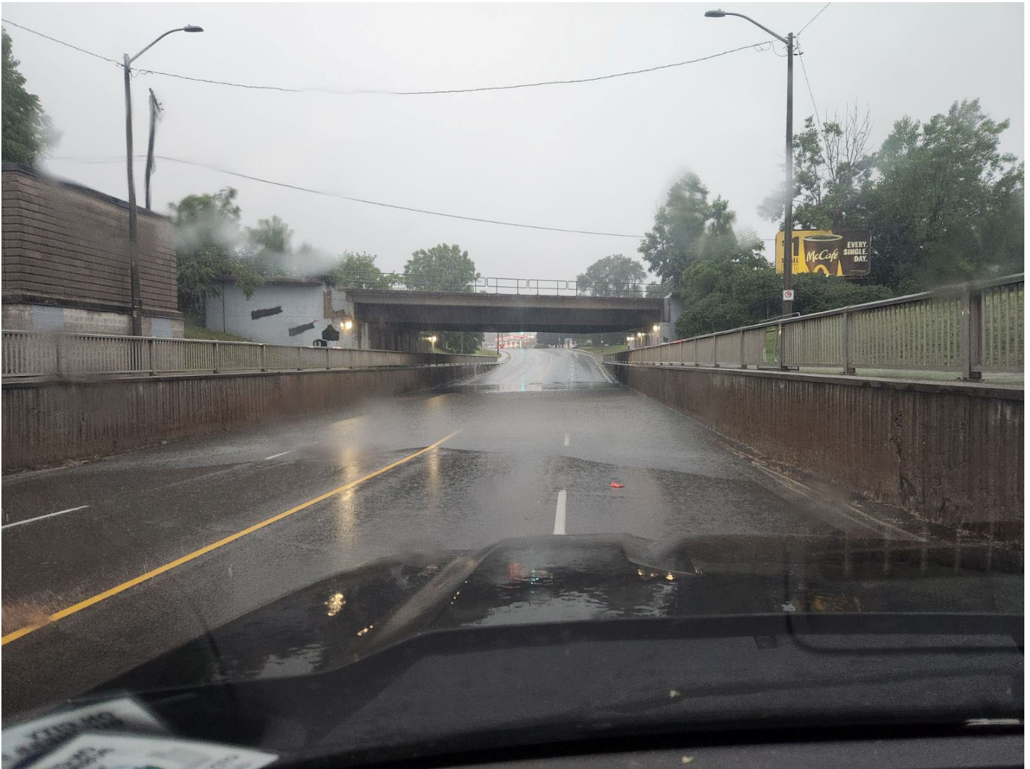
Figure 3: Cannifton Road rail underpass facing north (photo credit: City of Belleville)
