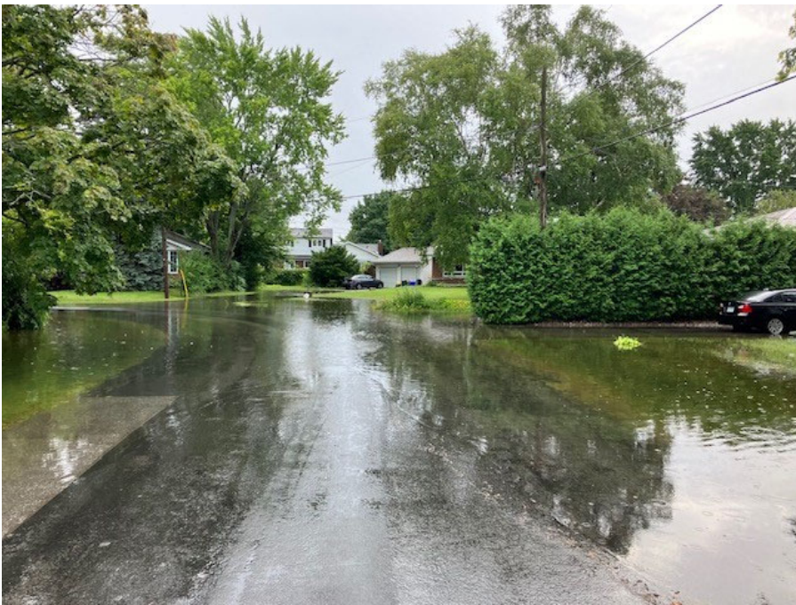
Figure 6: Ponding on local road and lawns in west end residential neighbourhood
